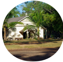
➤ St. Andrews Anglican Church at Angurugu, formerly an Anglican mission, then a township. This church has always been a peaceful meeting place.
