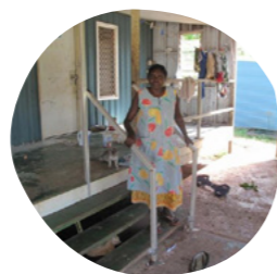
6 Rails installed at Joyce Lalara's Baniyala house. (2010)
